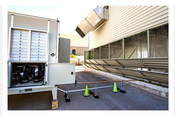
The Las Vegas Grand Prix installed an atmospheric water generator to capture water vapor exhaust from an existing evaporative cooling tower at the MGM Grand Hotel & Casino to help offset race-related water consumption.
